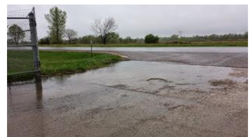
Standing water during a recent rain event
