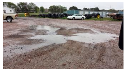
Standing water during a recent rain event
